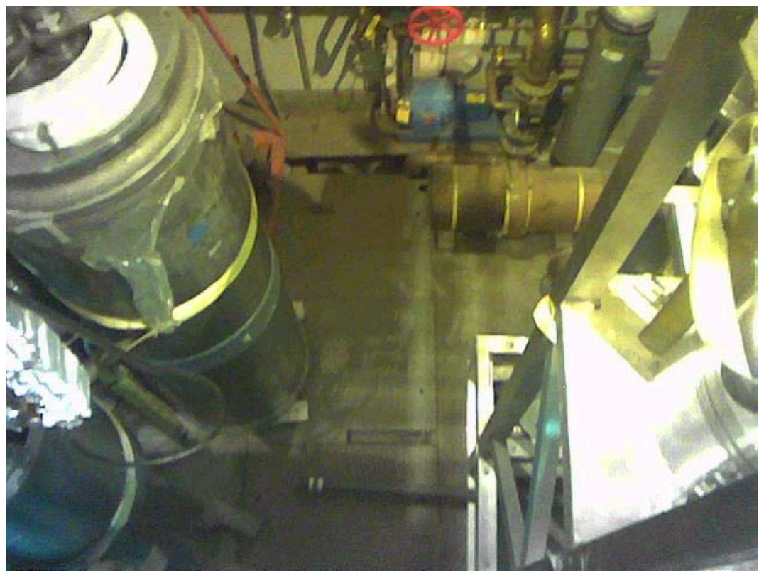
View looking down
